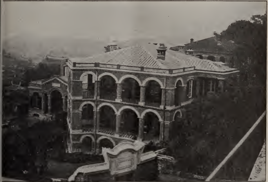
OPERATING PAVILION, DR. KINNEAR'S HOSPITAL, FOOCHOW CITY
